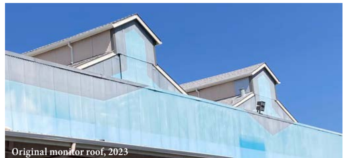
Original monitor roof, 2023
