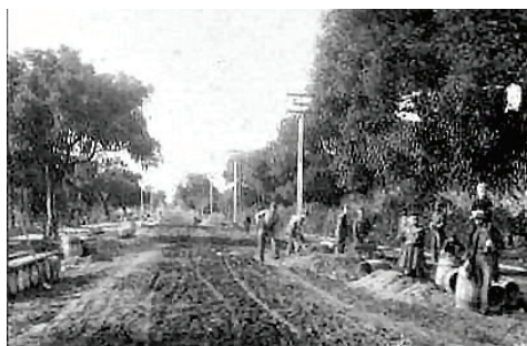
Waverley Street construction with Joseph Hutchinson in the foreground
