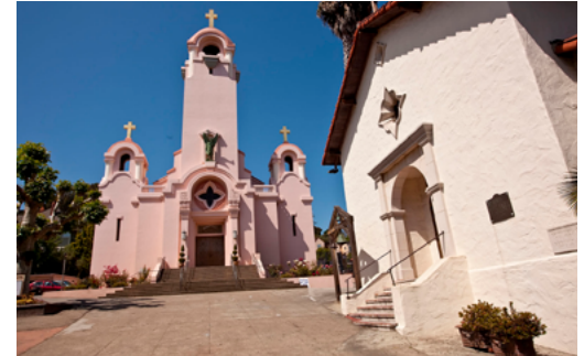
A replica of the original Mission San Rafael chapel, built in 1949, sits to the right of the current Saint Raphael's church. Courtesy of California Mission Resource Center.
